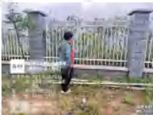
▲升压站厂界东 (8.15 昼间)
